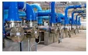
The SVAWPC receives secondary-treated effluent from the San Jose-Santa Clara Regional Wastewater Facility (RWF) and processes the secondary-treated effluent through three additional treatment processes (microfiltration, reverse osmosis, and ultraviolet light) to produce up to 8 million gallons per day of purified water. The purified water is blended with the recycled water supply produced at the RWF.
